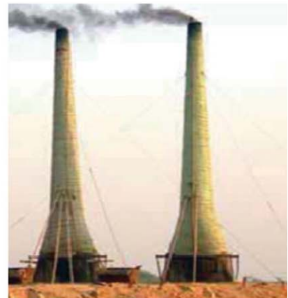
(b) Bull Trench Kiln (Movable chimney)
